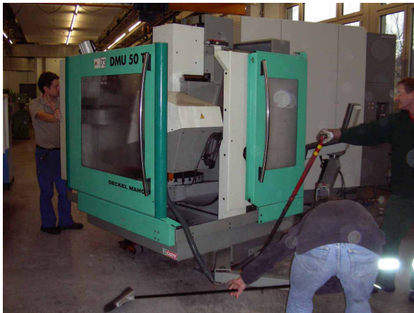
Figure 12.1: Installation of the new milling machine.
